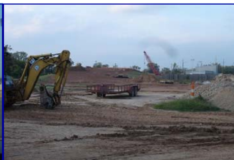
Benton Road Overpass Construction
