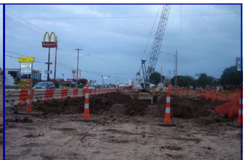
Youree Drive Construction
