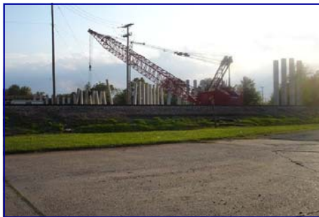
Benton Road Overpass
