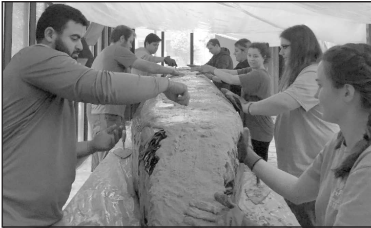
Placing the concrete onto the mold
