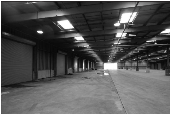
Figure 3. Photograph inside Shed 9. Note the bulkhead line running from foreground to rear door. Overhead clearance to the rafters from the bulkhead line is 17 ft 8 in
