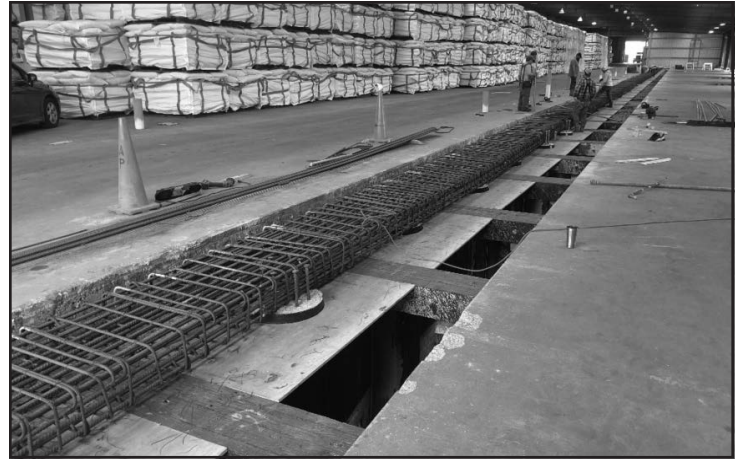
Figure 7. Concrete beam rebar layout prior to beam widening/bump-outs. Note out of tolerance helical pile in foreground
