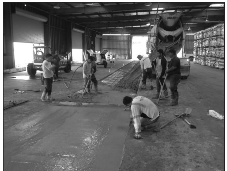
Figure 9. Finishing the topping slab
