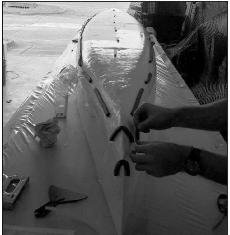
*Concrete Canoe progress: finished canoe mold being prepared for pour day*
